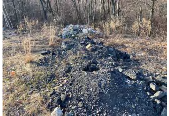
2. View of dumped materials along Haul Road.
