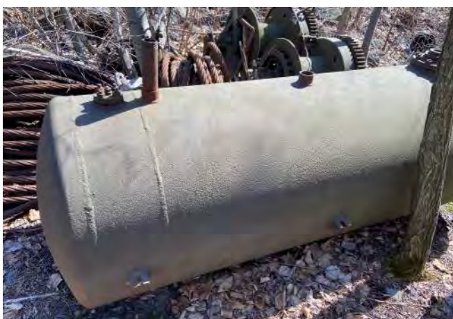
5. View of an empty storage tank on the eastern of the Site.
