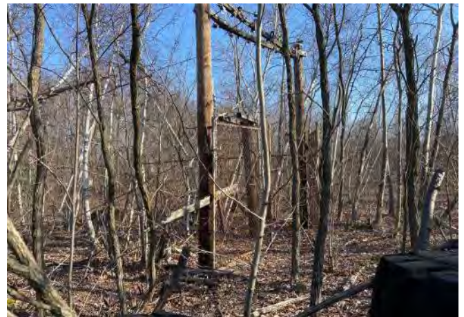
18. View of former fenced electrical station.
