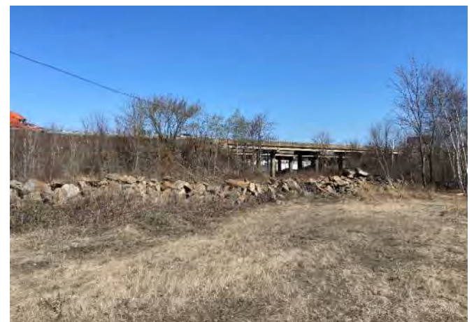
30. View of the northern portion of the Site.
