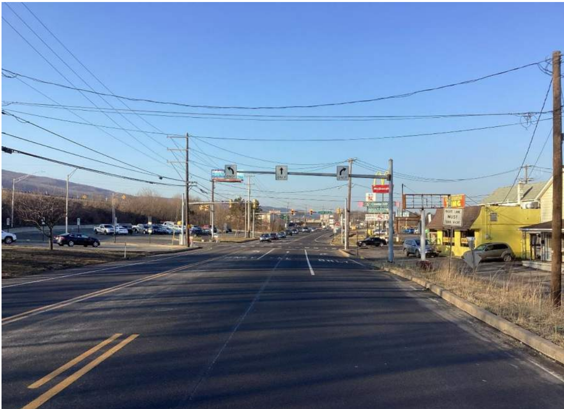
Direction / Road: Sb. Wilkes-Barre Township Blvd (SR 6309) Approach / Departure: Approach Distance: 150 Feet
