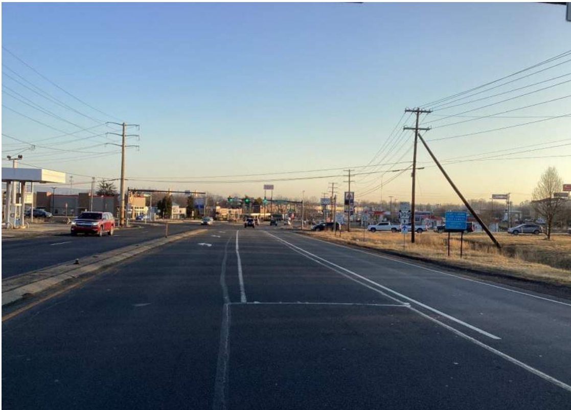
Direction / Road: Nb. Wilkes-Barre Township Blvd (SR 6309) Approach / Departure: Approach Distance: 150 Feet
