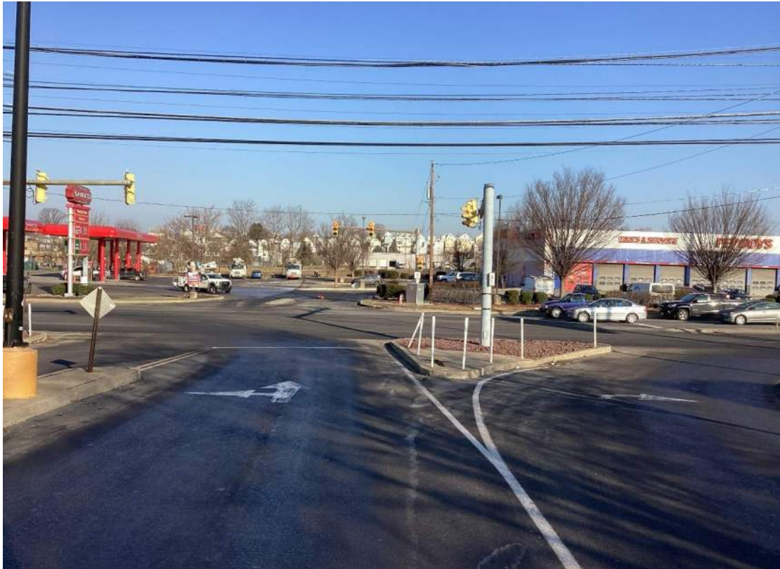
Direction / Road: Wb. Shopping Center Driveways Approach / Departure: Approach Distance: 50 feet
