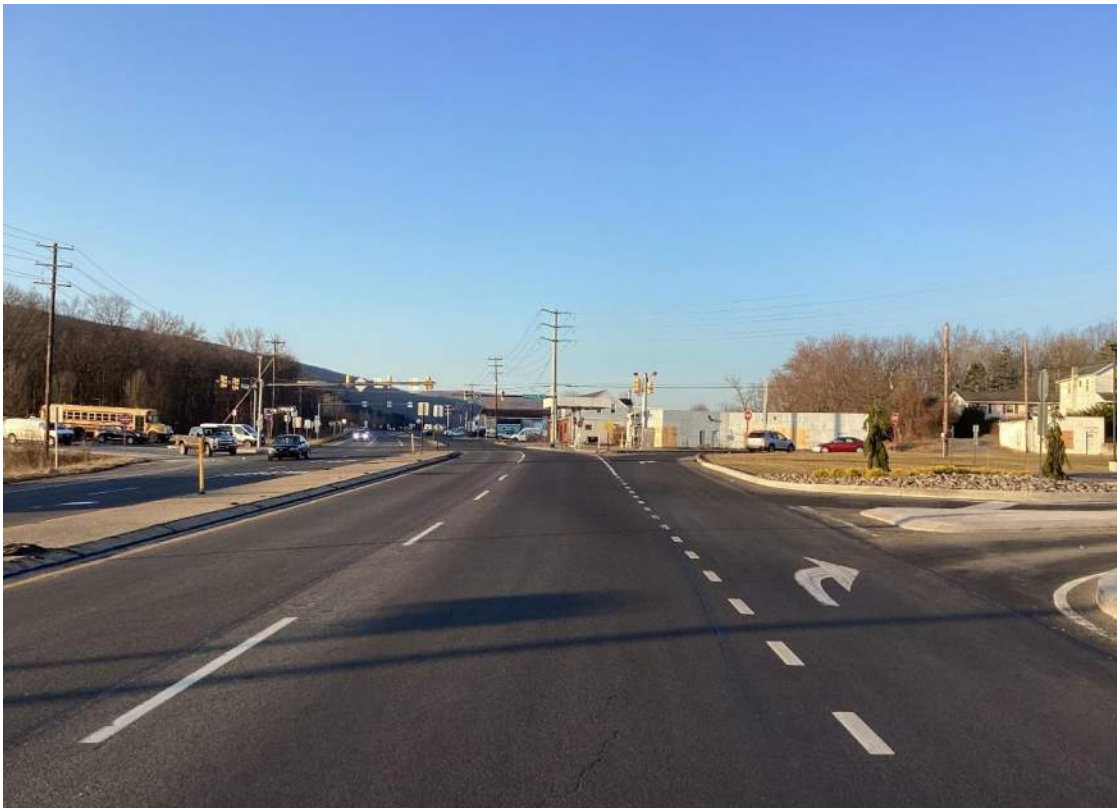
Direction / Road: Sb. Wilkes-Barre Township Blvd (SR 6309) Approach / Departure: Approach Distance: 150 Feet
